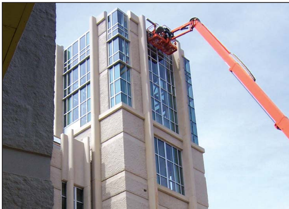
View from the concourse of one of the towers
