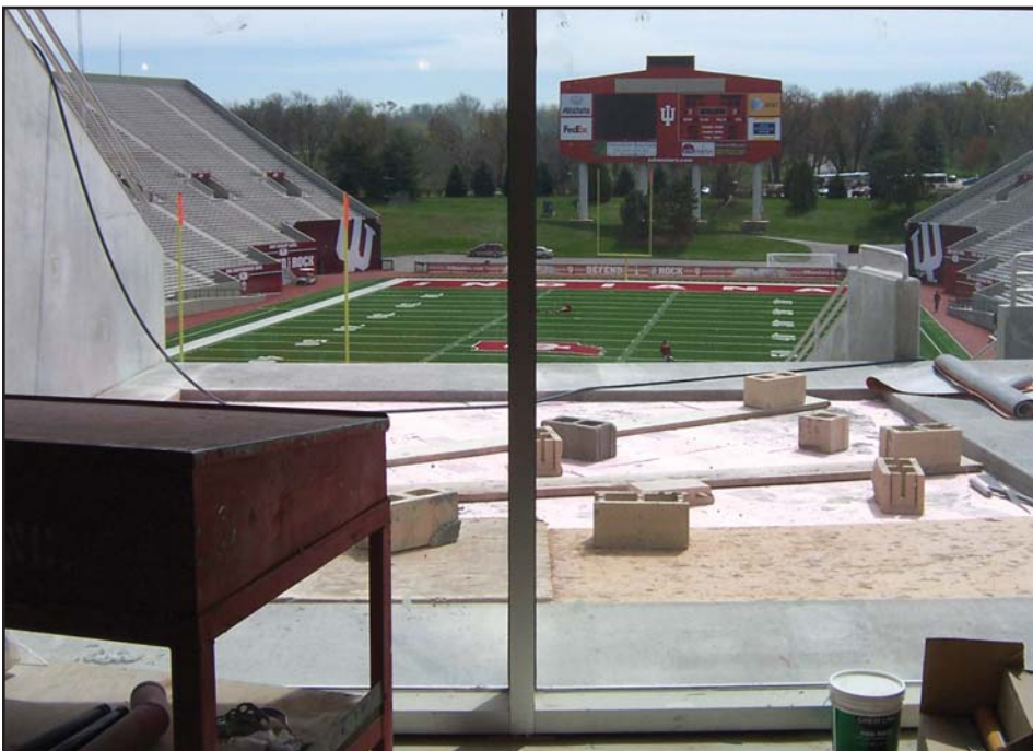
View from a coach's office overlooking the balcony
