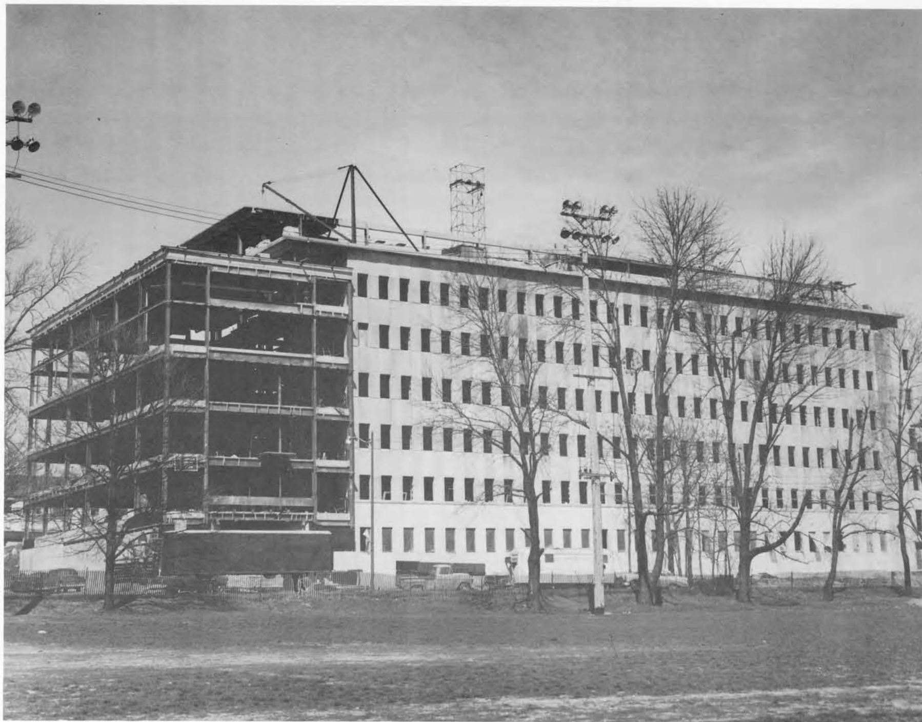
View of new Geology Building facing Tenth Street
