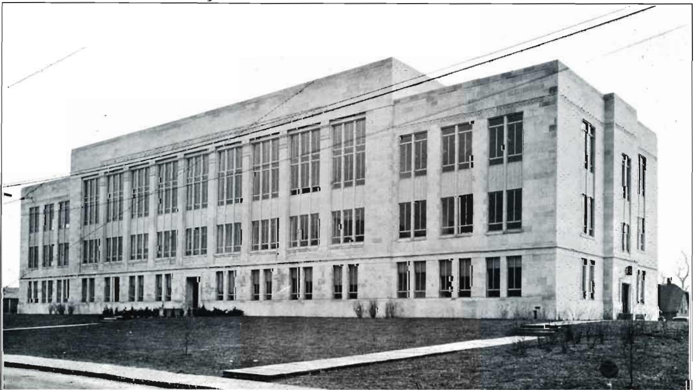
The new I.U. School of Dentistry building, completed in 1933.
